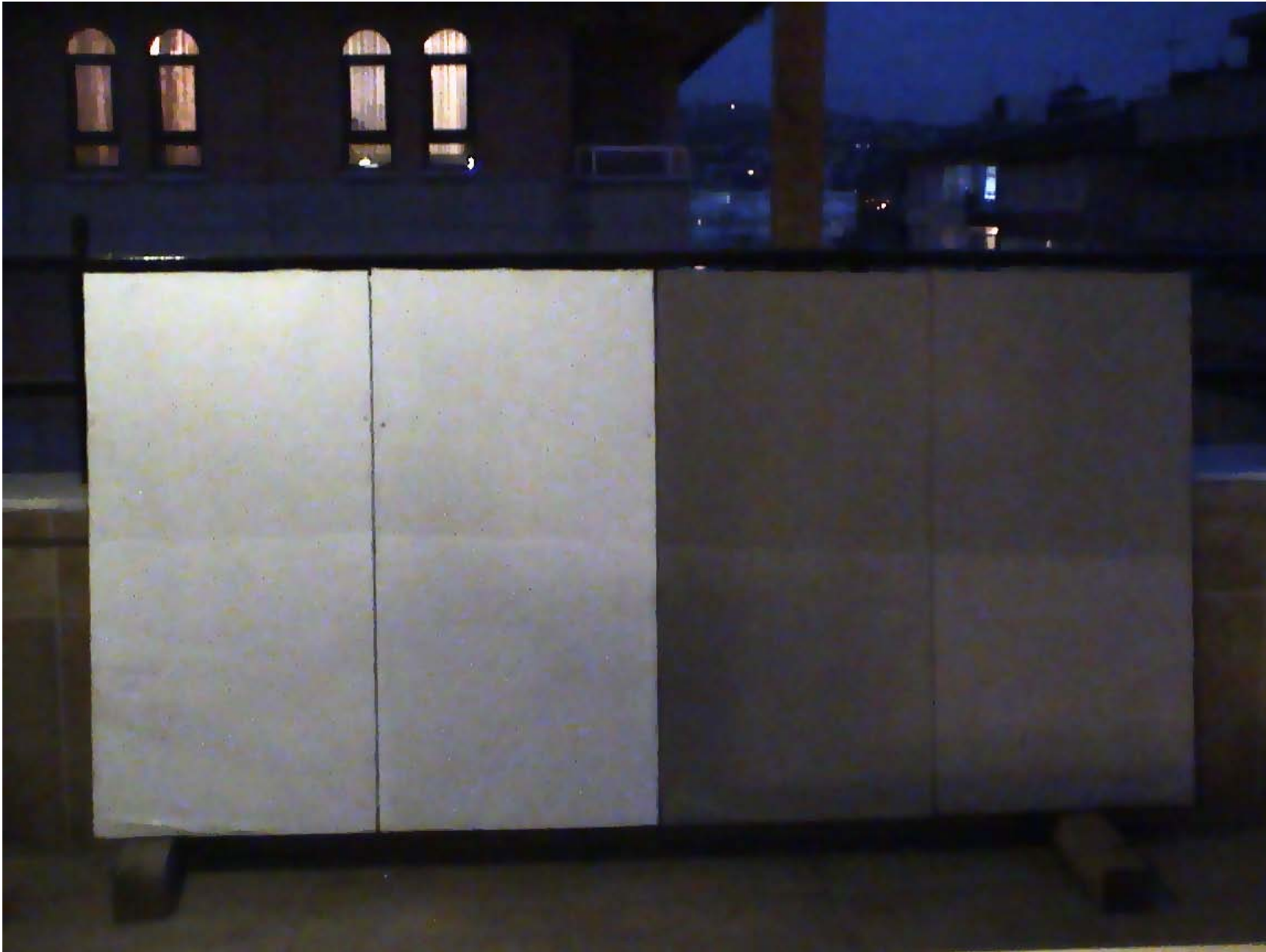
Photo 7: Showing all four nano-reinforced paint coated surfaces. With half of them later coated with regular paint to show the contrast.
